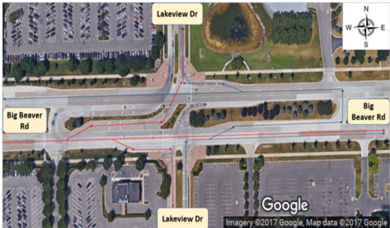
Figure 2- Existing Superstreet Intersection in Troy, MI (Red and blue lines show the routes of EB, and NB, respectively. WB, and SB follow the same pattern. Source of aerial: Imagery ©2017 Google, Map data ©2017 Google)
